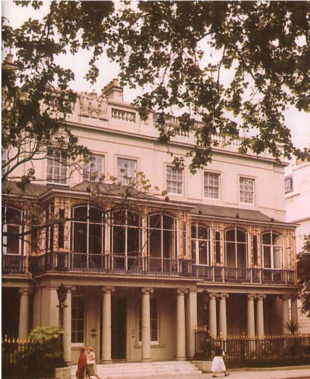
Dudley House, Park Lane: Mid 19th century conservatory addition
