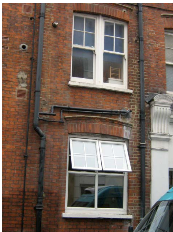
Replacement windows, although improving thermal performance, can harm character and appearance of buildings.
